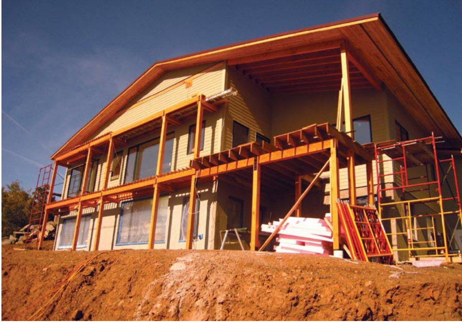
Roof overhang and a trellis structure manage the solar gain.
