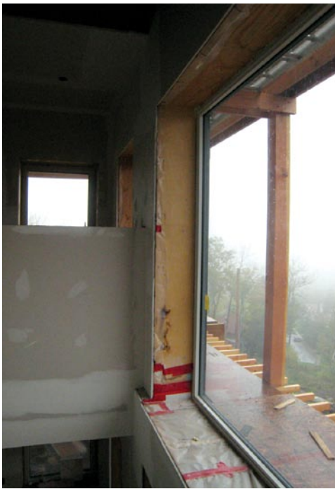
Insulated fiberglass window frames with triple-pane glazing allow solar gain and prevent heat loss.
